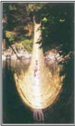
Figure 6.7 : Rope Bridge (Arunachal Pradesh)
