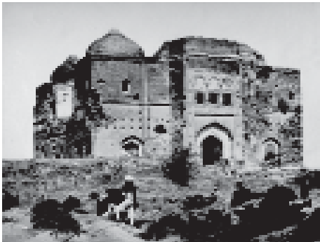
Fig. 11.8 A mosque on the Delhi Ridge, photograph by Felice Beato, 1857-58 After 1857, British photographers recorded innumerable images of desolation and ruin.
